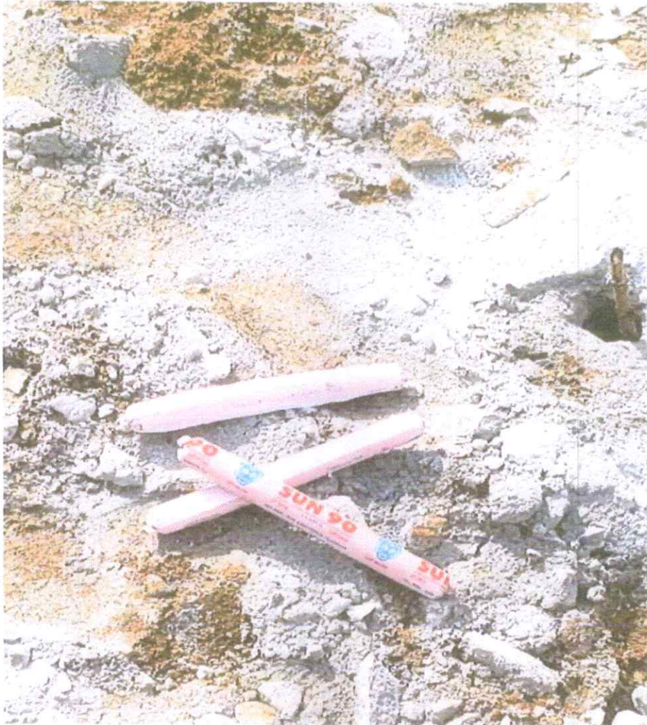
FIG. 6 A VIEW OF EXPLOSIVES USED IN THE QUARRY
