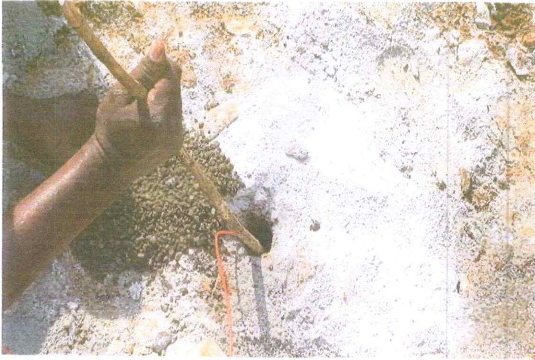
FIG. 9 STEMMING OF BLASTHOLES
