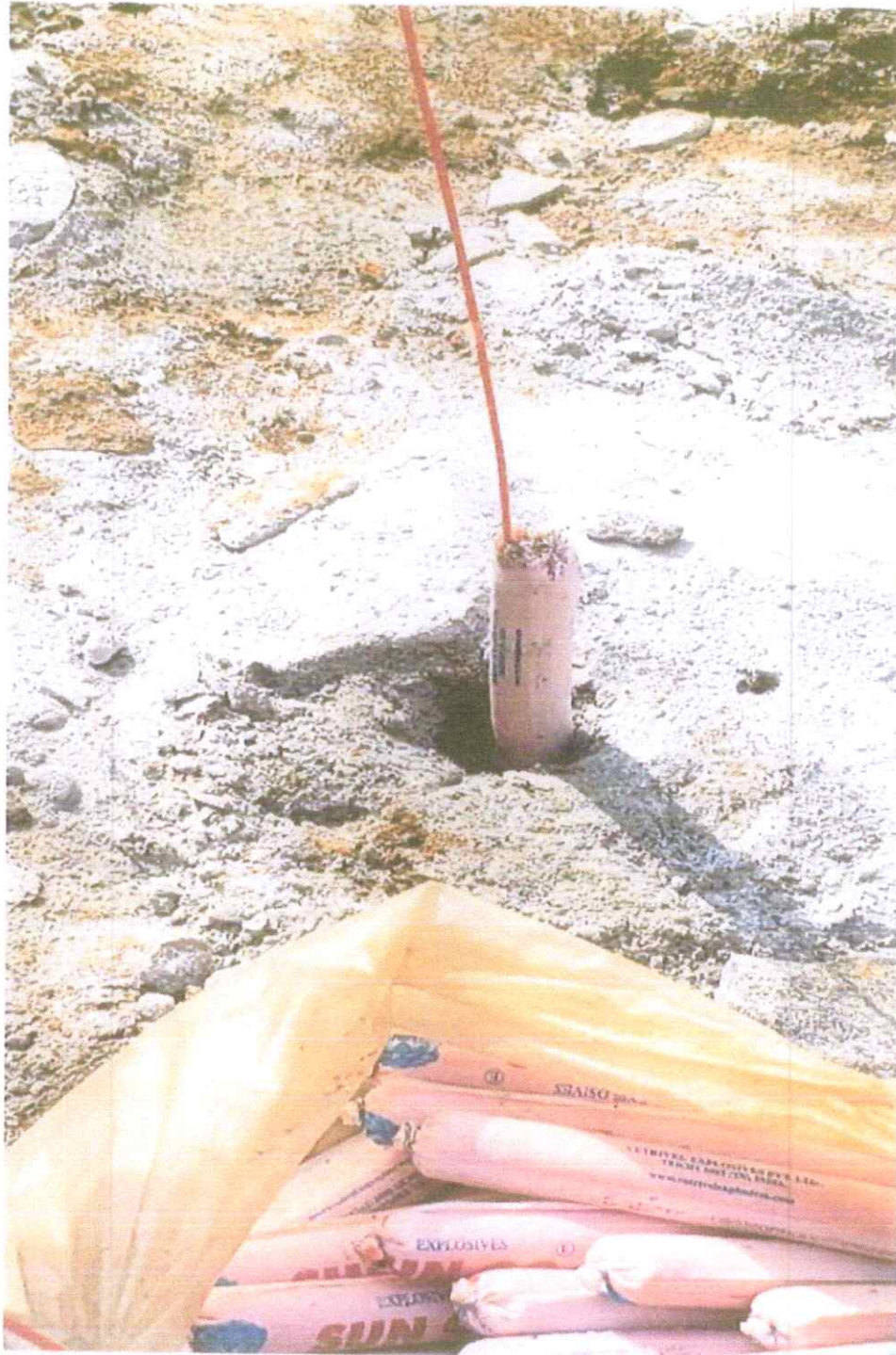
FIG. 8 CHARGING OF BLASTHOLES
