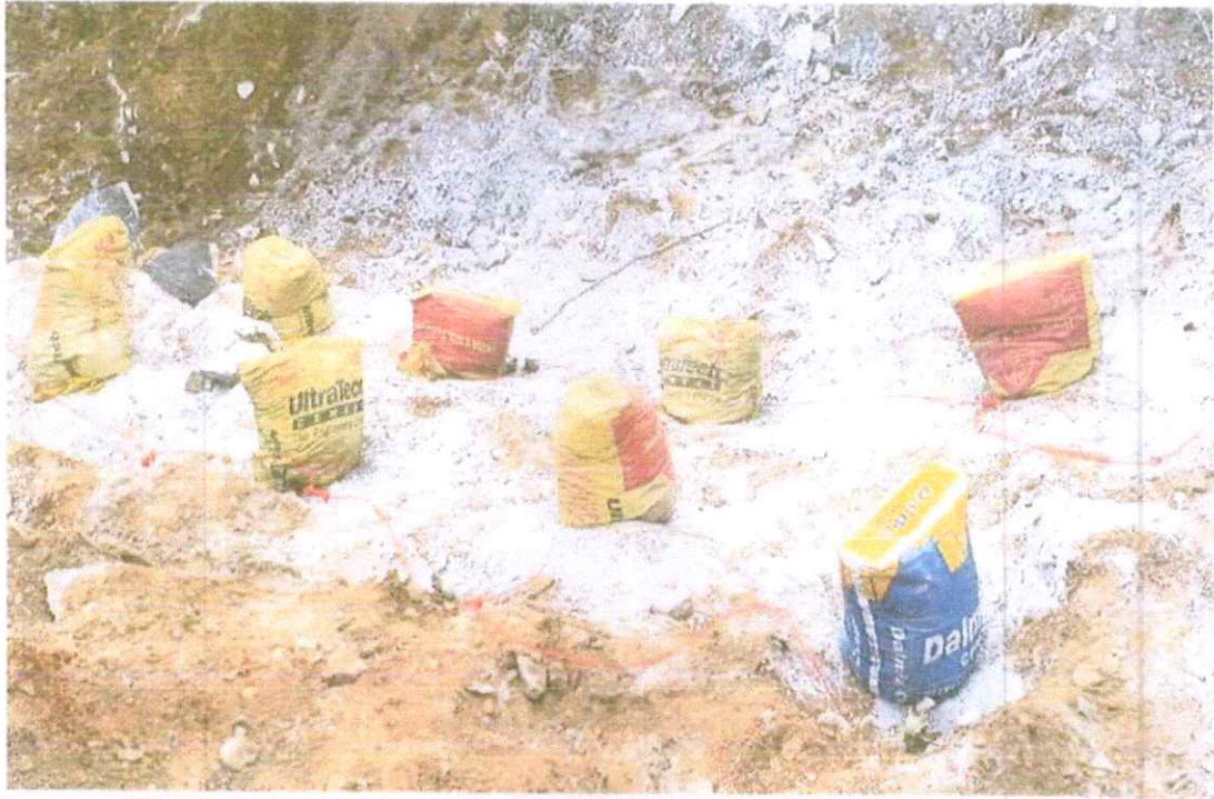
FIG. 11 MUFFLING ARRANGEMENT WITH SAND BAGS OVER THE BLASTING AREA
