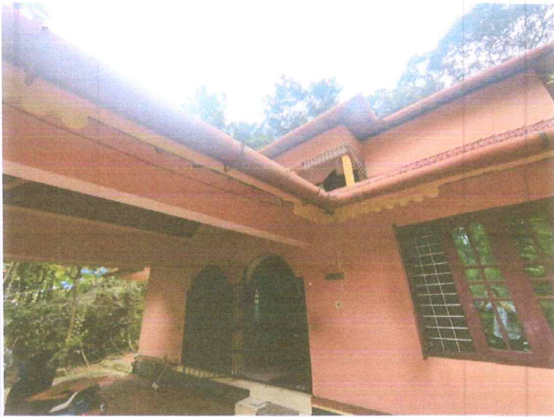
FIG. 3 A VIEW OF THE HOUSE INSPECTED BEFORE THE BLAST
